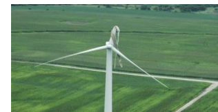
Wind Blade Damage by Heavy Storm
